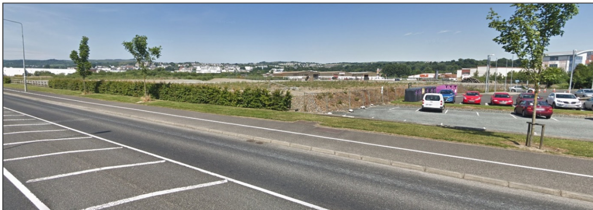
Plates 2.7 and 2.8: Google Street View image of the proposed site
